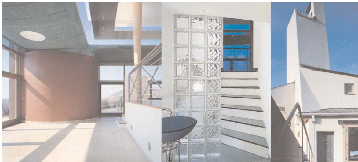
images below from left: Windows in living room retract fully into the floor to open interior to the outside; Chimney passively ventilates the house; Stair leading into bathroom
